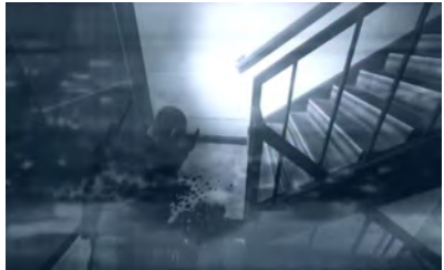
Abb. Condemned30 (SCU Building)
